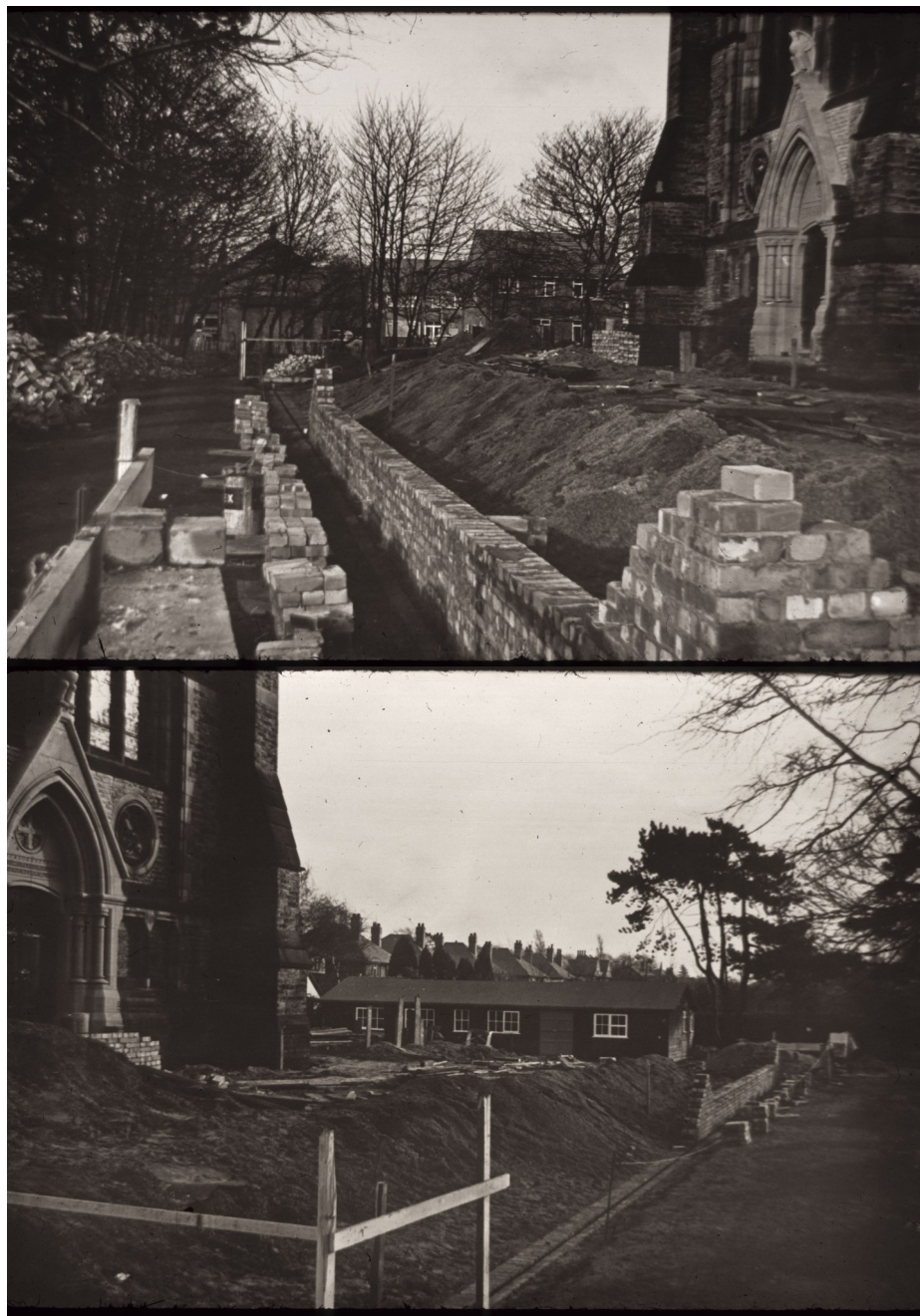
Some photographs of the hall construction courtesy of Tim Marlow.
